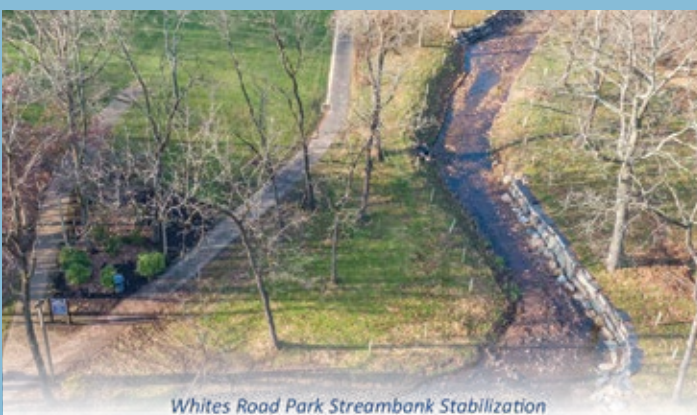
Whites Road Park Streambank Stabilization
